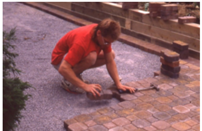
Almost done – pavers are going down, retaining wall is going up.
