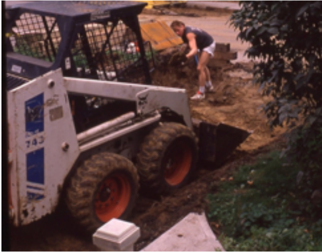
The 'Bob Cat' and Ambrose – excavating the driveway.
